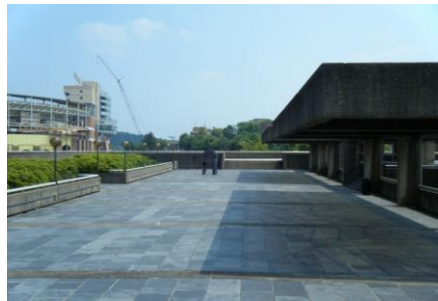
South Facing View
