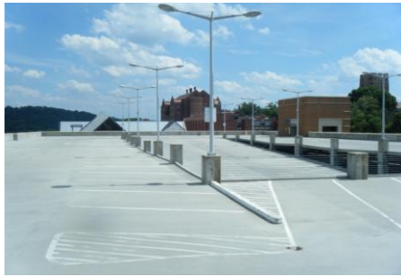
South Facing View
