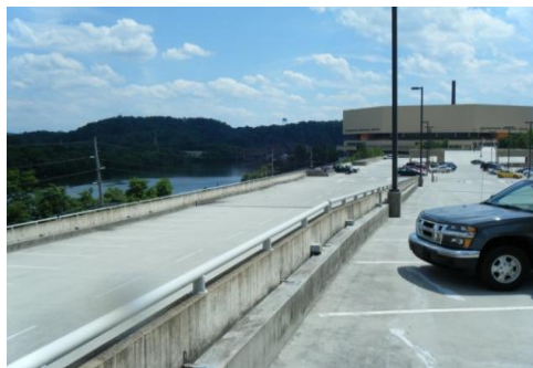
South Facing View
