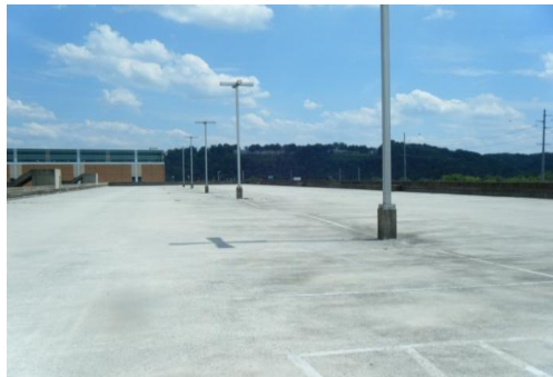
South Facing View
