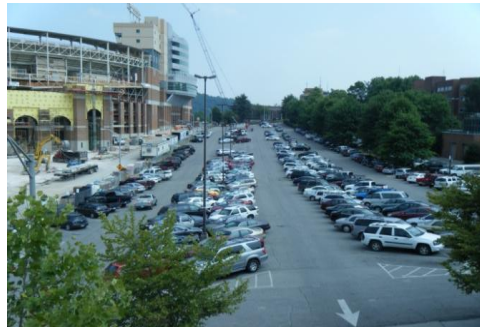
South Facing View
