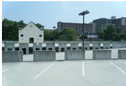
South Facing View
